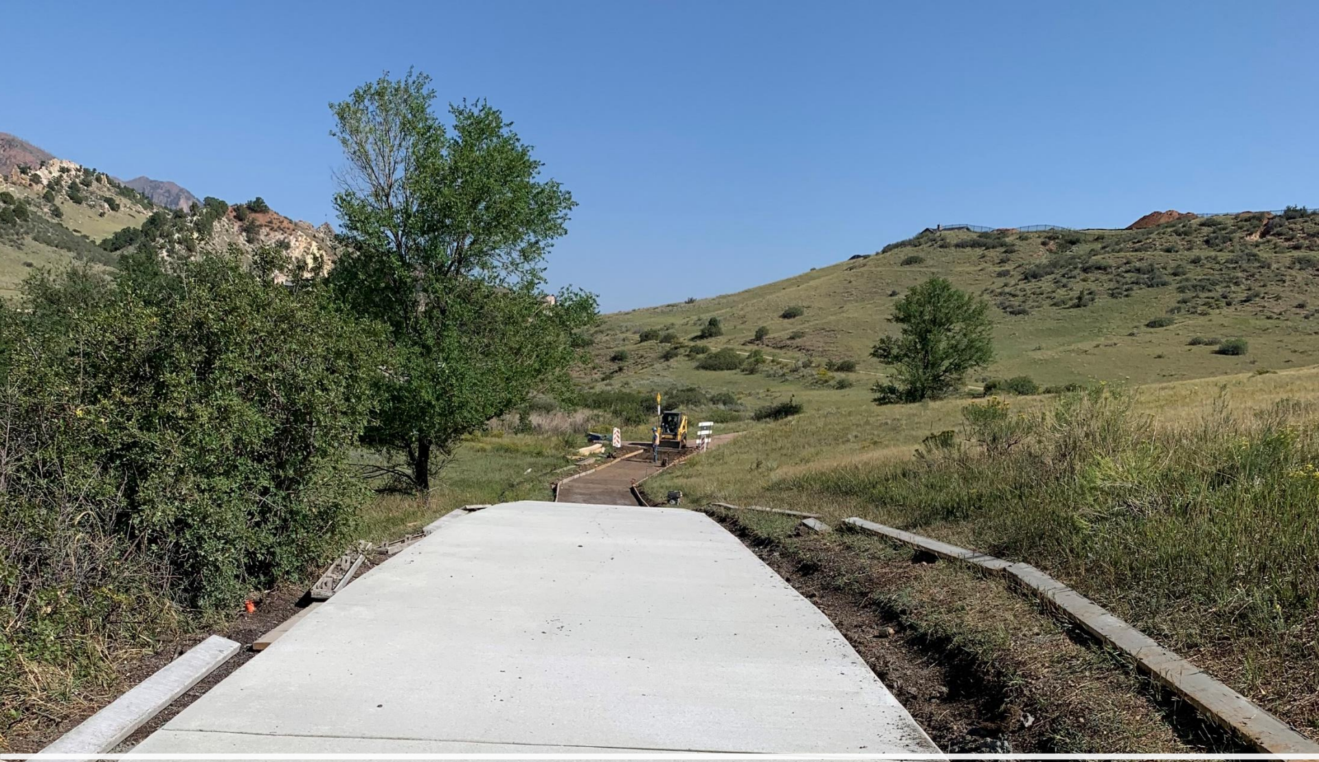
Palmer Mesa Trail-under construction
