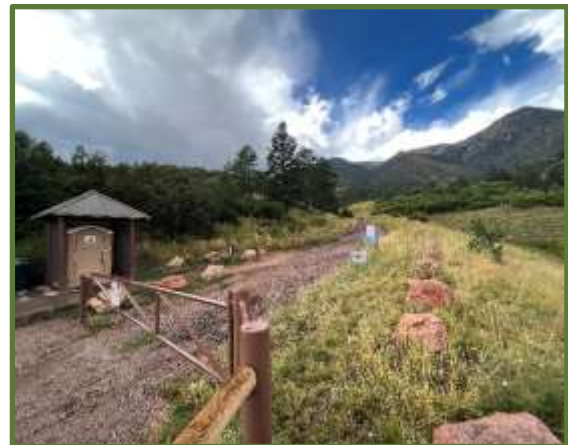
Utilities access road looking west
