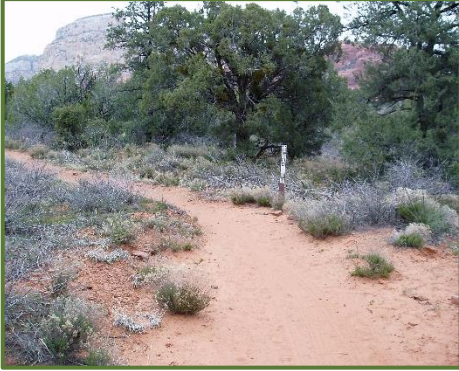
active closure with smooth transition to reroute trail section, proper signage and intentional closure of illegal trail with obliterated trail, water diversions, and intentionally placed branches.
