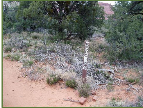
active closure with smooth transition to reroute trail section, proper signage and intentional closure of rogue trail with obliterated trail, water diversions, and intentionally placed branches.
