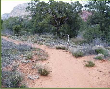
active closure with smooth transition to reroute trail section, proper signage and intentional closure of rogue trail with obliterated trail, water diversions, and intentionally placed branches.
