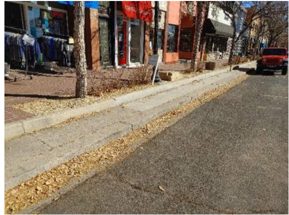
Figure 12. Double Curb in Old Colorado City
