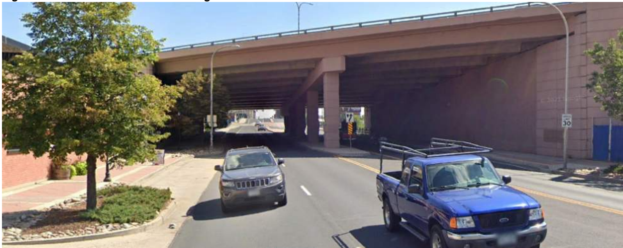
Figure 29. Colorado Avenue Looking West Under I-25
