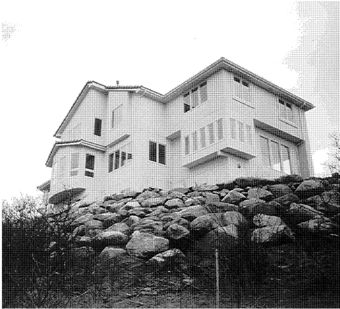
House inappropriately placed on fill platform.
