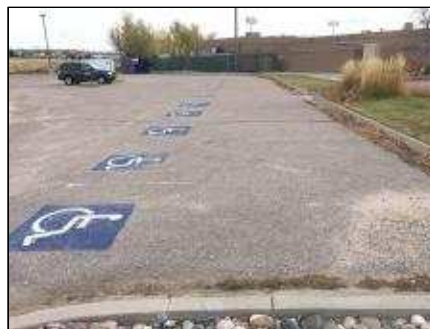
Accessible parking is not compliant
