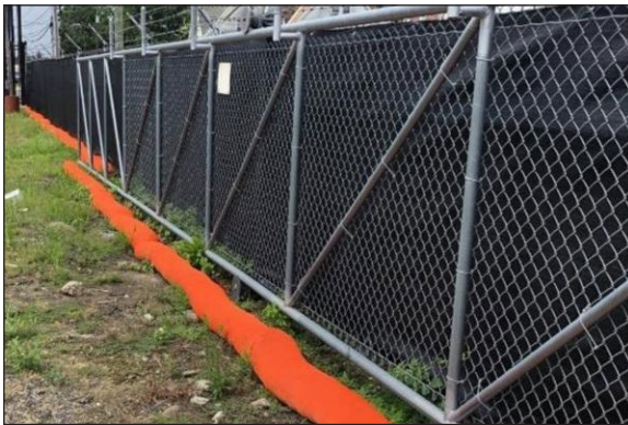
Filtrexx SiltSoxx EXTREME used in rugged conditions.
