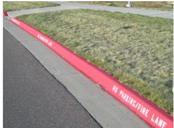
Figure 15 - Typical fire lane striping installation
