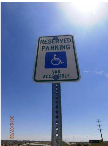
Image of noncompliant signage at accessible parking
