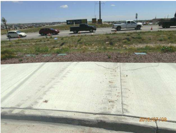
Image of fractured sidewalk
