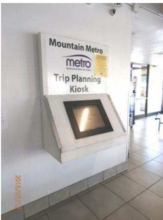
Image of trip kiosk projecting into path
