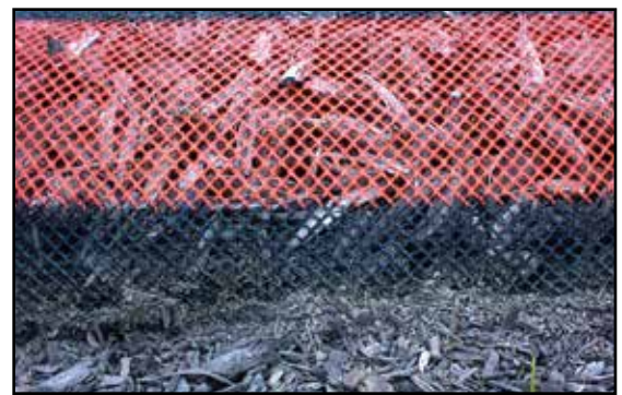
Close Up of Sediment Control
