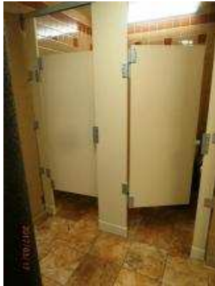
Finding 184833 Additional Photo
