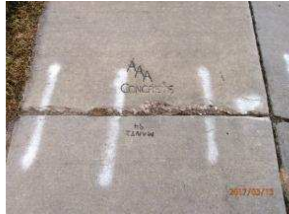
Finding 184829 Additional Photo
