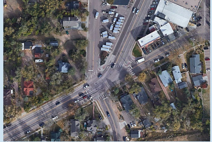
Existing intersection of South Tejon Street, Cascade Avenue, Ramona Avenue, and Cheyenne Boulevard currently includes five approaches to a single point. The City of Colorado Springs is reconstructing the intersection into a modern roundabout.
