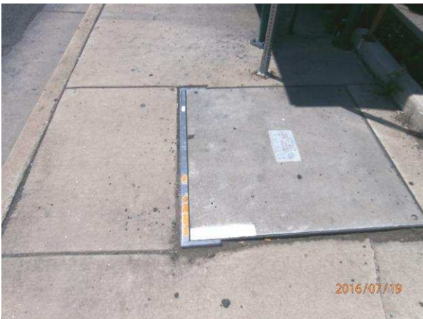
Image of vertical displacement in sidewalk
