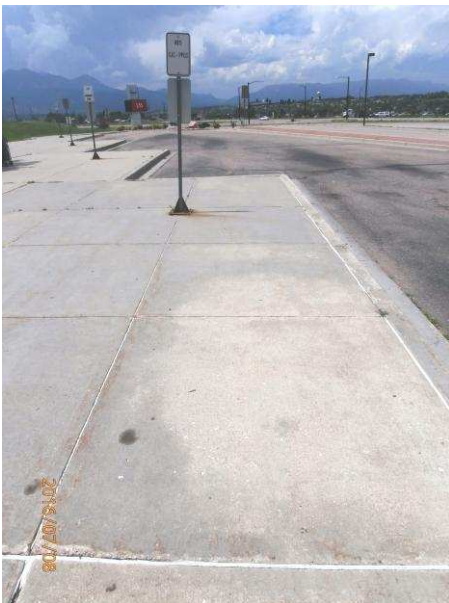
Image of sidewalk with excessive running and cross slopes
