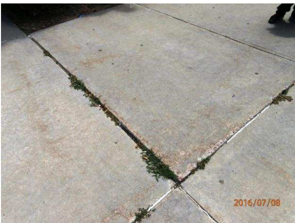
Image of gaps and vertical displacement in sidewalk.
