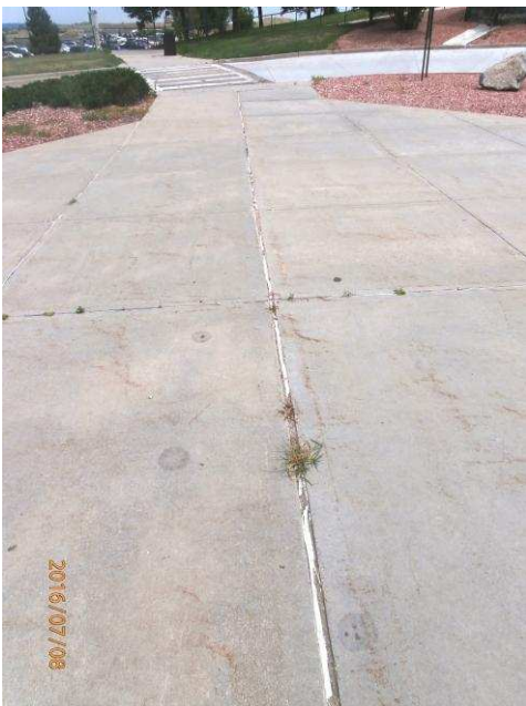
Image of gap in sidewalk
