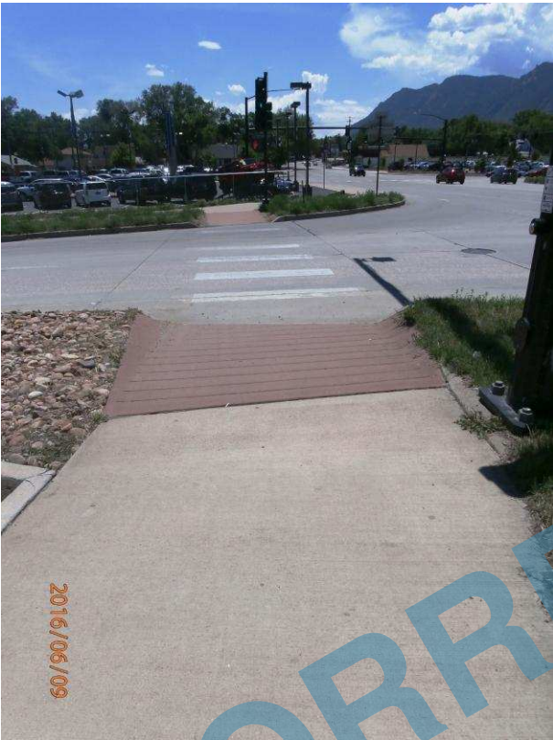
Image of curb ramp without detectable warnings
