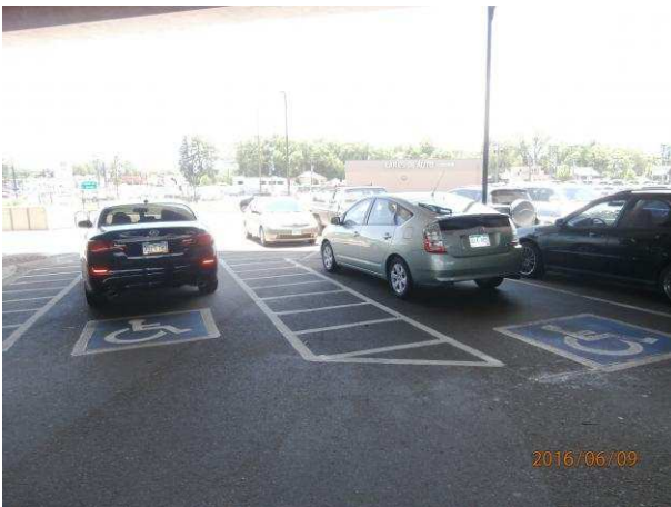
Image of narrow access aisles
