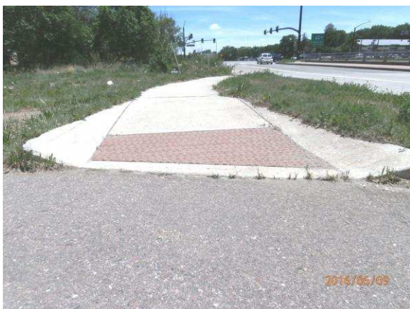
Image of vertical displacement at curb ramp
