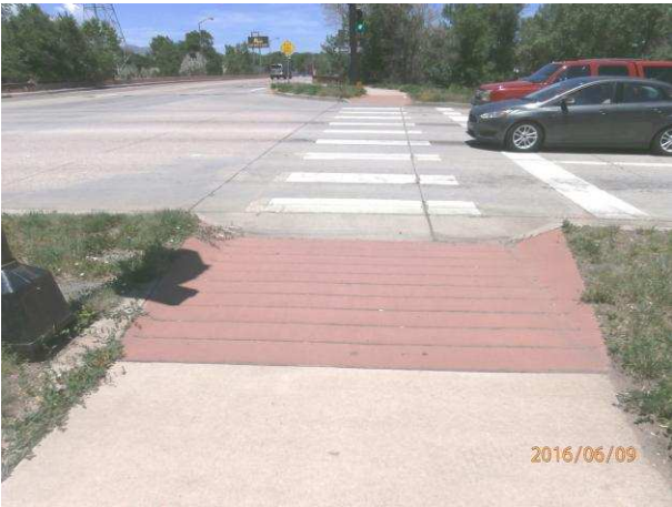
Image of curb ramp without detectable warnings
