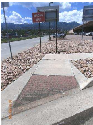
Image of vertical displacement at curb ramp
