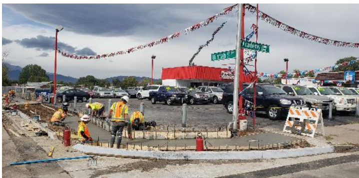
Public Right-of-Way Construction
