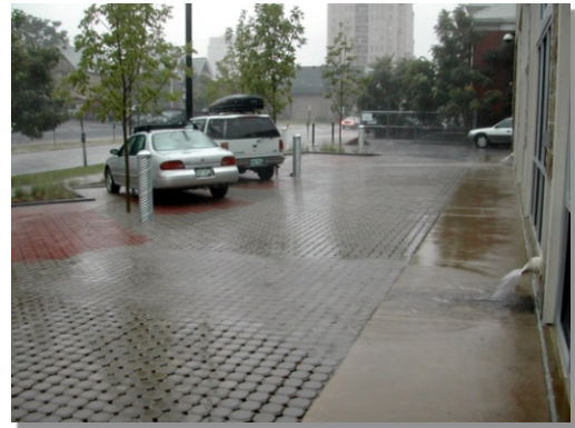
Photograph 1-1. Permeable Pavement. Permeable pavement consists of a permeable pavement layer underlain by gravel and sand layers in most cases. Uses include parking lots and low traffic areas, to accommodate vehicles while facilitating stormwater infiltration near its source. Photo courtesy of Bill Wenk.
