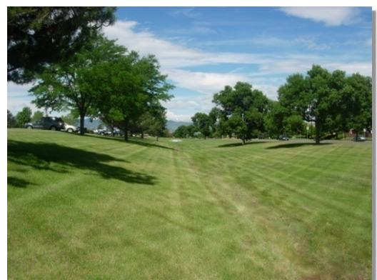
Photograph 1-3. Grass Swale. This densely vegetated drainageway is designed with channel geometry that forces the flow to be slow and shallow, facilitating sedimentation while limiting
