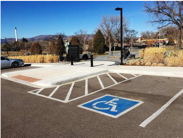
Image of accessible parking without signage
