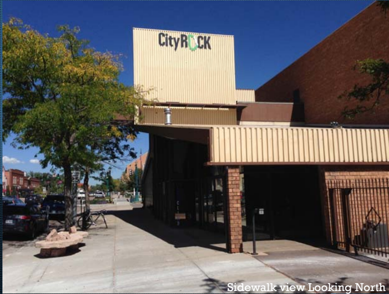
Sidewalk view Looking North
