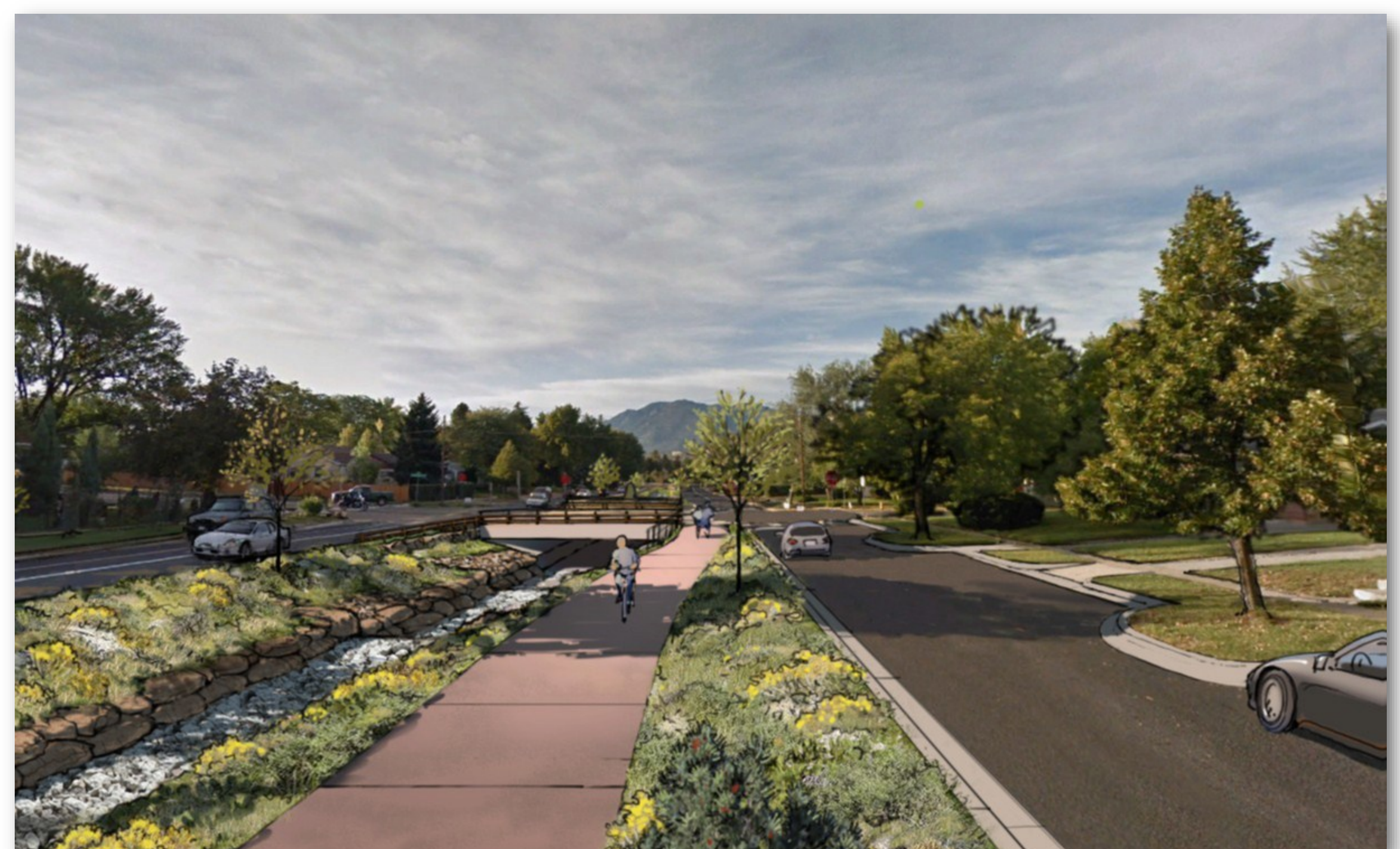
Grass and rock-lined channel and multi-use trail along 31st Street
