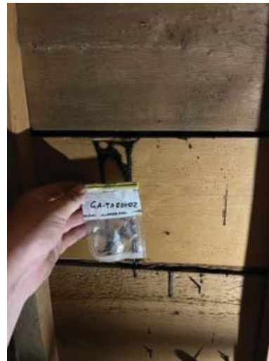
Sample: GA-TAR01-02 Result: None Detected
