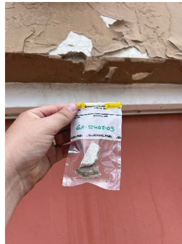
Sample: GA-STU02-04 Result: 2% Chrysotile
