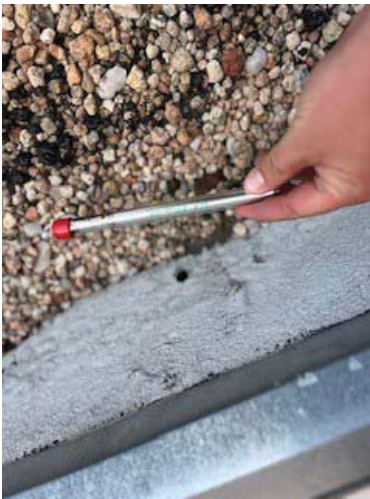
Sample: GA-RFL01-02 Result: 60% Chrysotile in brown felt
