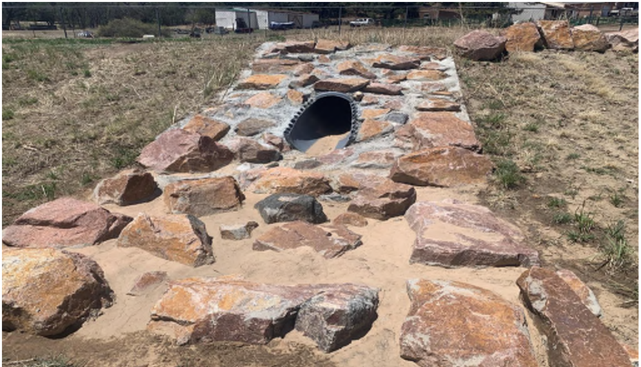
Field Inspection Completed by: Trent Davis, HDR, Inc
