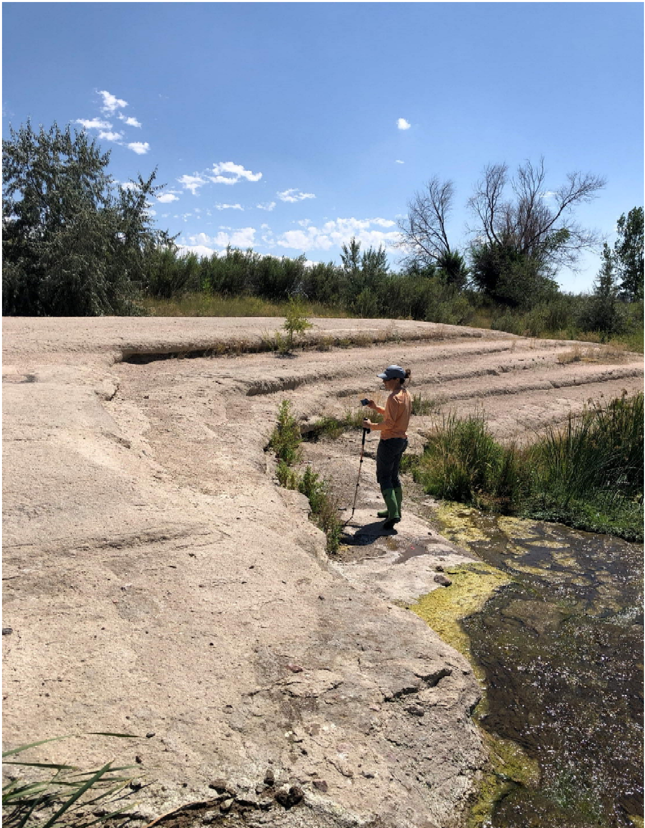
PHOTO AREA 4 - EXISTING CONDITIONS OF EAST SIDEWALL - LOOKING EAST
