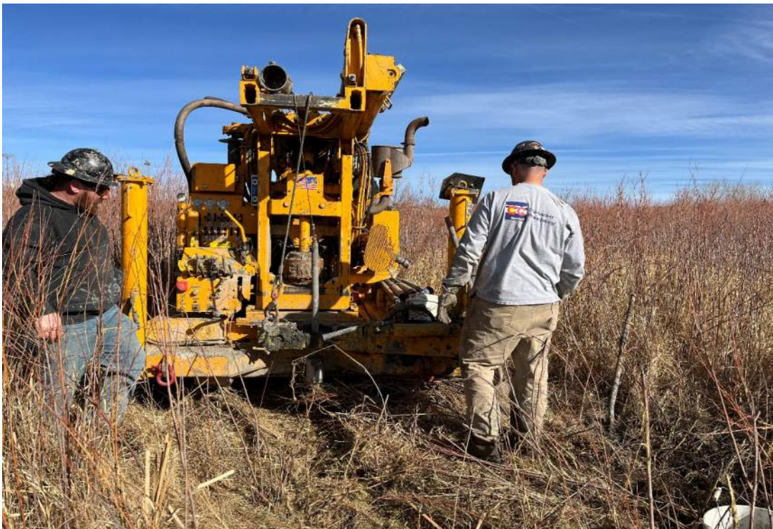
DRILLING BORING B-3 - LOOKING NORTH - JANUARY 2022
