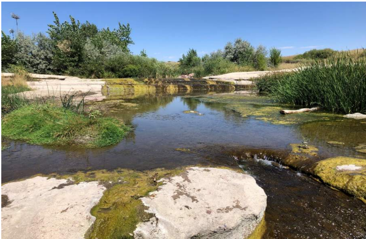
EXISTING DROP STRUCTURE - LOOKING NORTH
