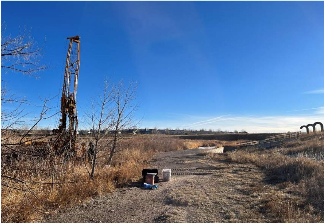
DRILLING BORING B-1 - LOOKING EAST - JANUARY 2022
