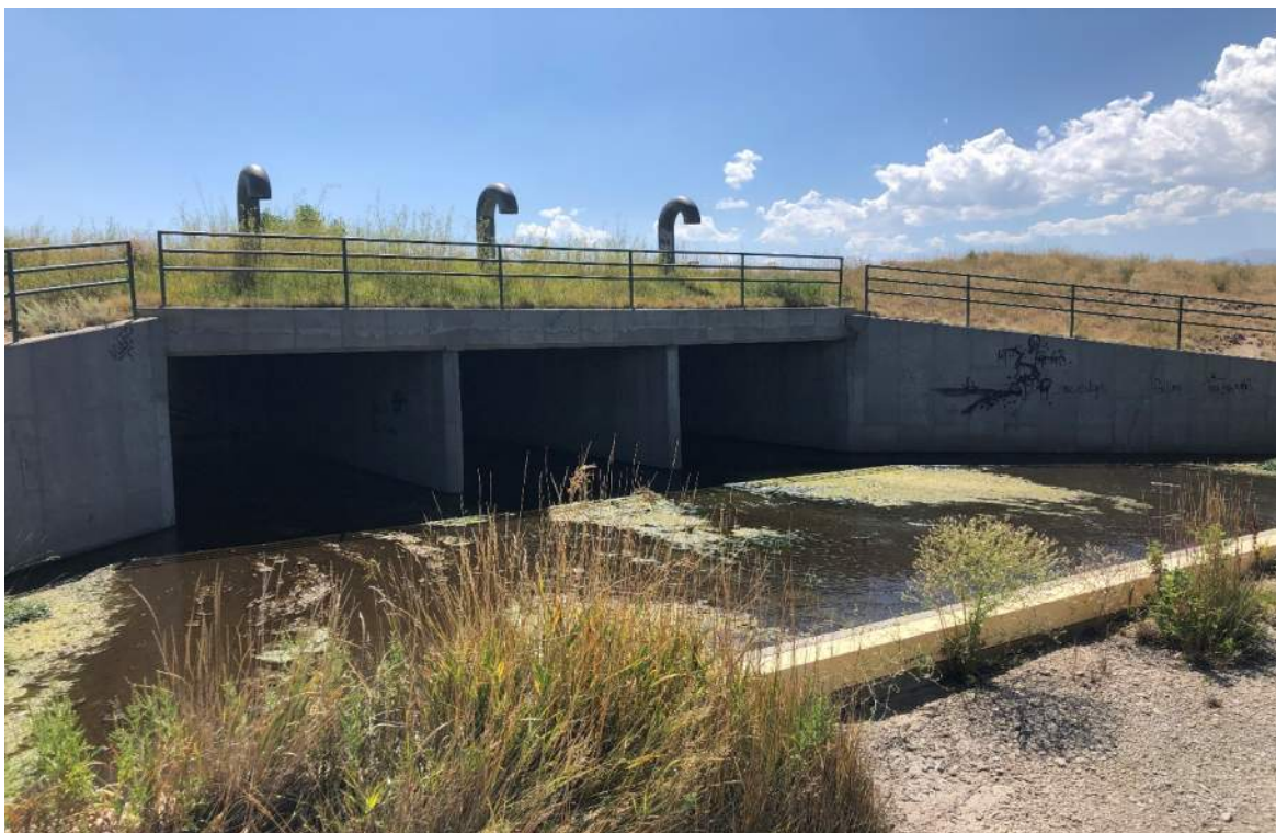
EXISTING OUTLET STRUCTURE - LOOKING SOUTHWEST - AUGUST 2021
