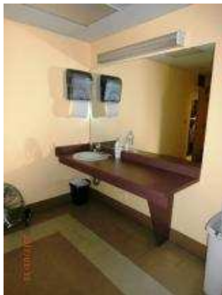
Finding 184789 Additional Photo
