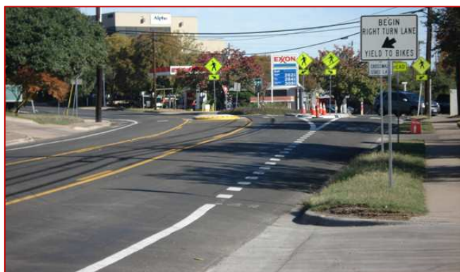
Figure 9: Improvements at Balcones and Parkercrest Drive.
